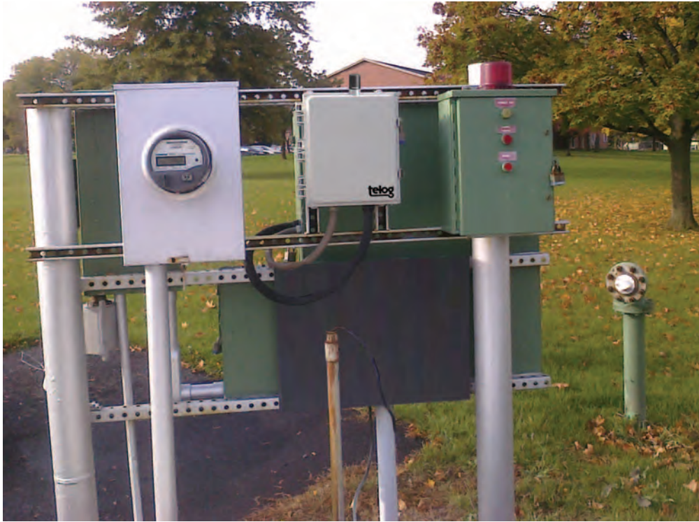
RS-33u monitoring a lift station
