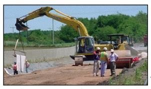
FMC's onsite Eastern Surface Impoundment (ESI). The affected areas of the ESI were then graded, capped with clean soil and revegetated.
