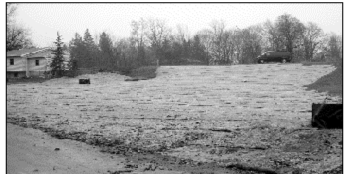
Culvert 105 (Margaret Droman Park)
